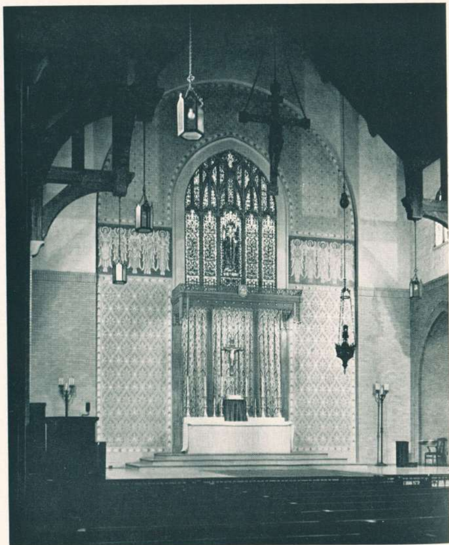
THE SANCTUARY AFTER RENOVATION IN 1946
