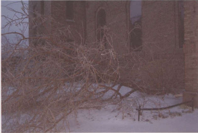
Tree snapped at base near east transept entrance.
